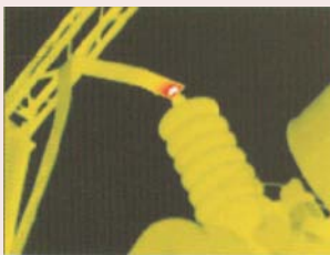
Transformer connector Abnormity
