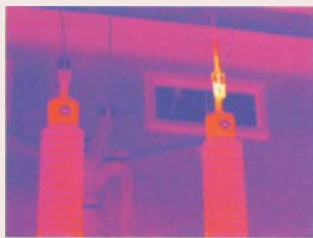
Axis Connection Overheat
